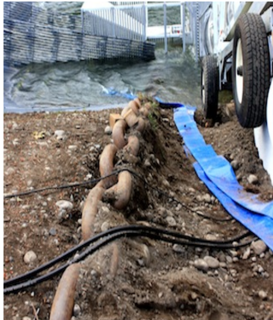
Figure 17. The Nisqually Weir anchor chain substrate rail. Photo courtesy of Nisqually Indian Tribe.
